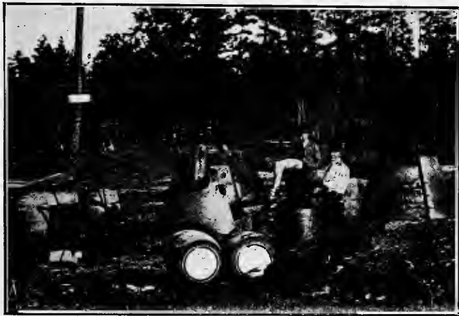
Fig. 14. Distilling Stumps in Place
